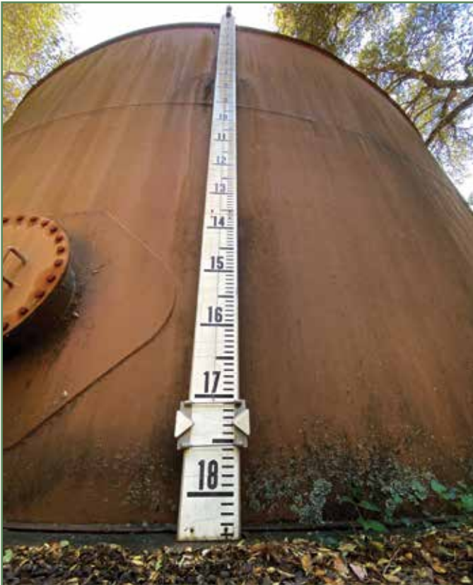
Filoli's 150,000 gallon domestic water tank at full capacity
